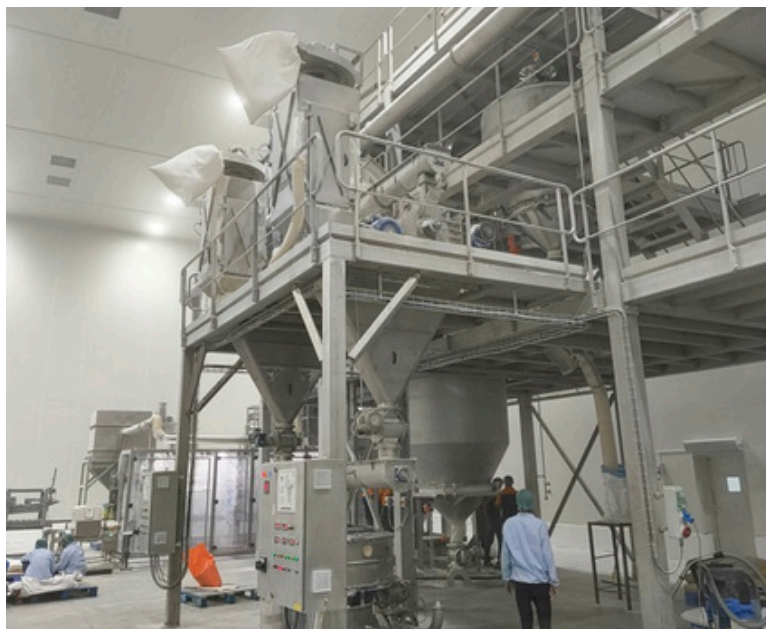
► Installation of 2 Nos. DP® CNT-320PD CONTRA Pin Mill in West India
